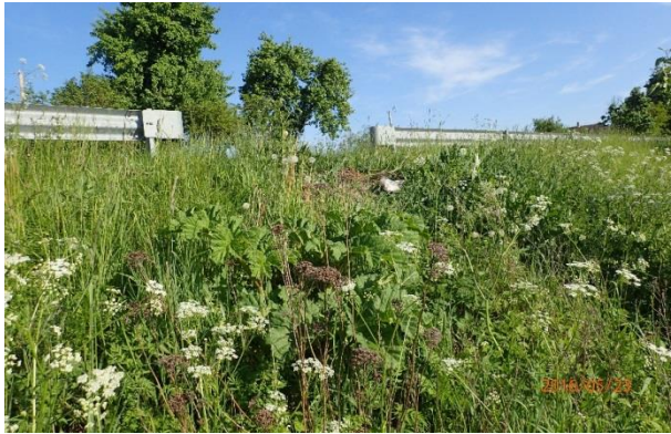
Fig 3.12 a) Before treatment, May 2016
